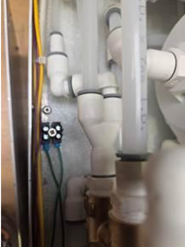
Leakage sensor Block terminal, black with 2 green cables
